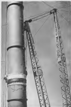
WELDER LAMPE climbs aloft, cuts lashings after lift. WELDER LAMPE ta subi na laria, pa corta cablanan.
